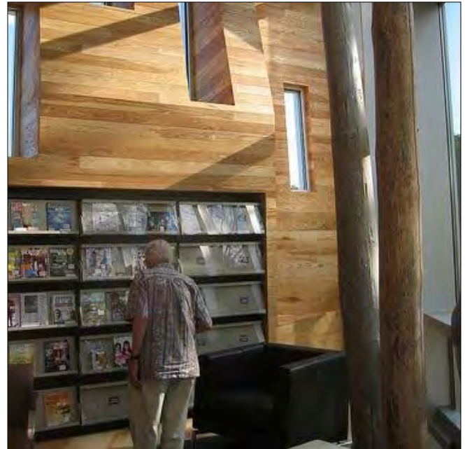
The new Traverwood Branch of the Ann Arbor District Library features extensive use of ash wood as flooring, paneling, and beams. The wood came from emerald ash borer-killed trees harvested from the development site prior to construction.
